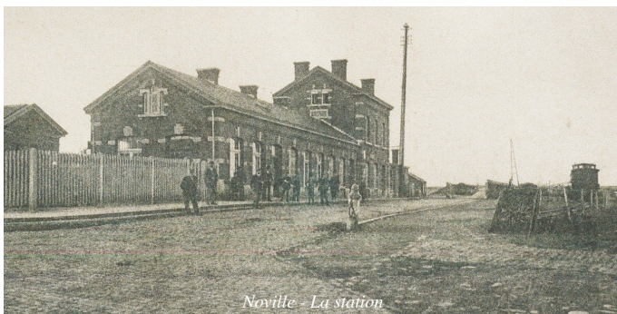
Noville - La station
